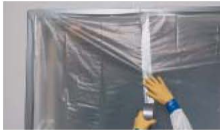
Hanging and Splicing Poly Fig.032 3M™ Duct Tapes can be used in many containment applications. The wider widths provide extra holding power for large, heavy sheets.
